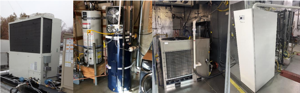
Figure 16: Commercial/Prototype FFHPs in GTI Energy Demonstrations: Engine-driven VRF, Sorption-type Water Heater, Sorption-type Whole House Combi System, and Thermal Compression-type Heat Pump Boiler (Source: GTI Energy)
