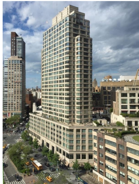
Figure 47: High-rise Building in New York City [Source: Mfr B]
