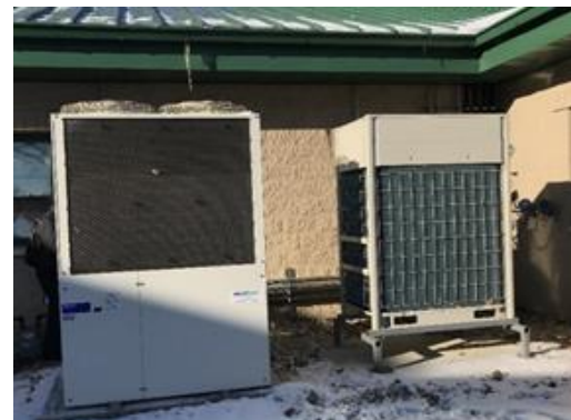
Figure 17: Side-by-side Comparison of FFHP and CCHP Solutions in 2020 [Rowley, 2020]
