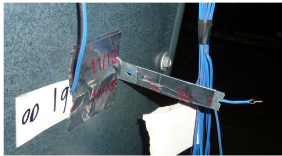
Figure C11. Typical Thermocouple Temperature Measuring Device Mounting
