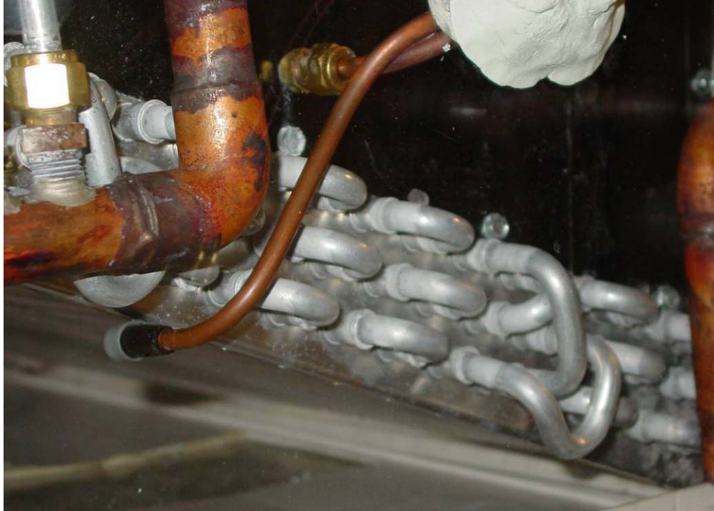
Figure 4.2 Static pressure taps used to measure air side pressure drop through lower slab
