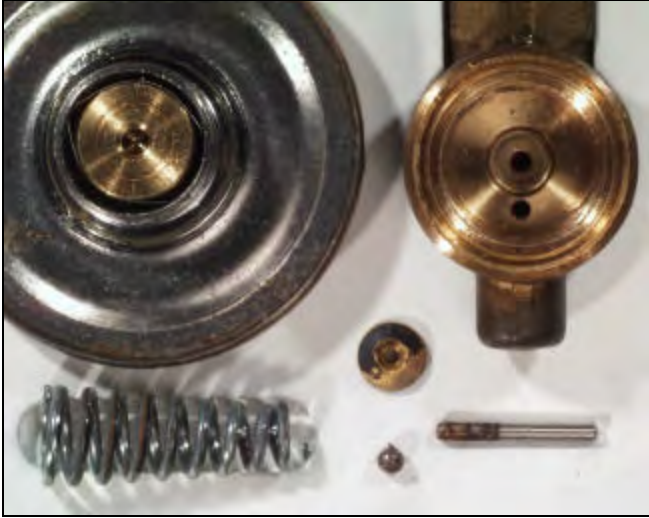
Constant Pressure Expansion Valve (macro)
