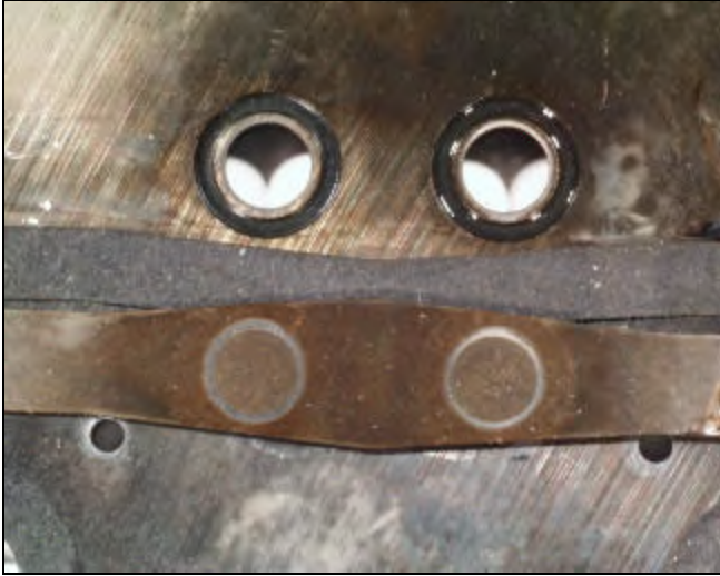
Valve Plate and Reed/Discharge (macro)
