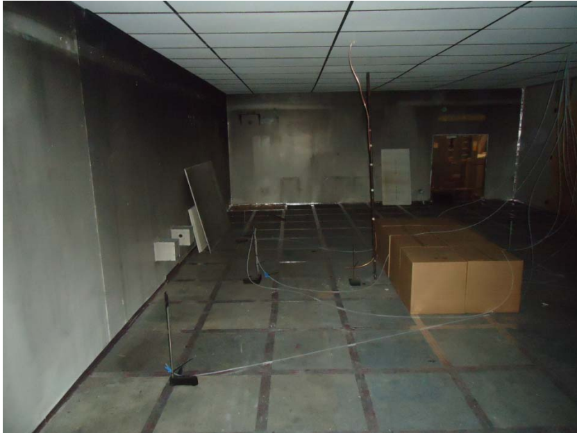
Inside Garage Facing East
