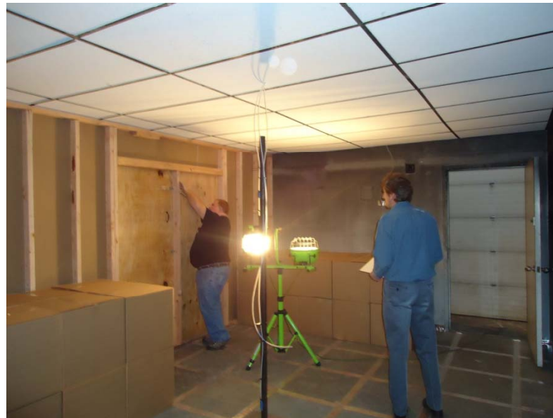
Inside Kitchen – Facing East
