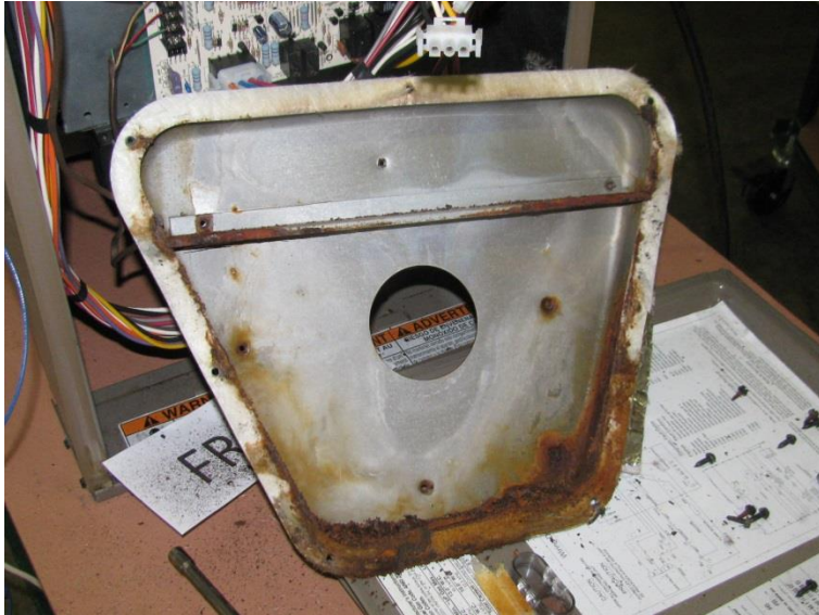
Collector Box Removed Showing Vestibule Panel Behind Collector Box
