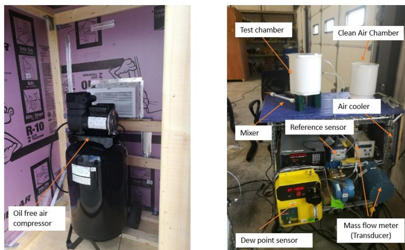
Figure 1-3. Pictures of the Test Facility
