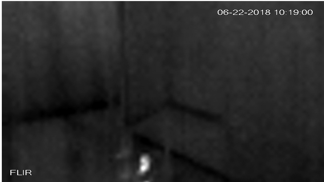
Figure 398 – RI_05 Small flaring at the location A electric arc.
