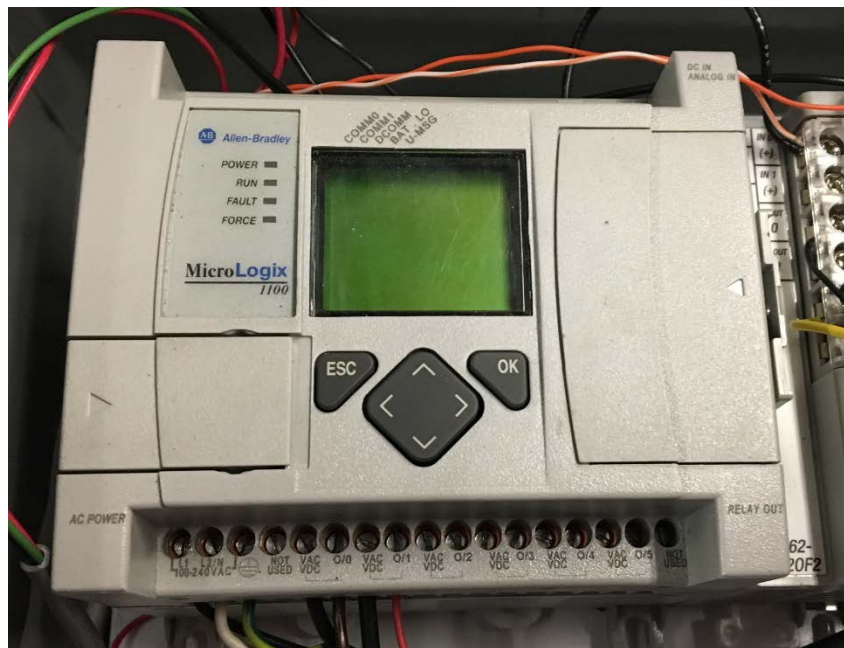
Figure 596 – Mass Flow System Programmable Logic Controller (PLC)
