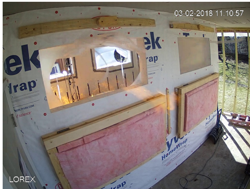
Figure 126 – CP_08 Flame extension through the west side vent
