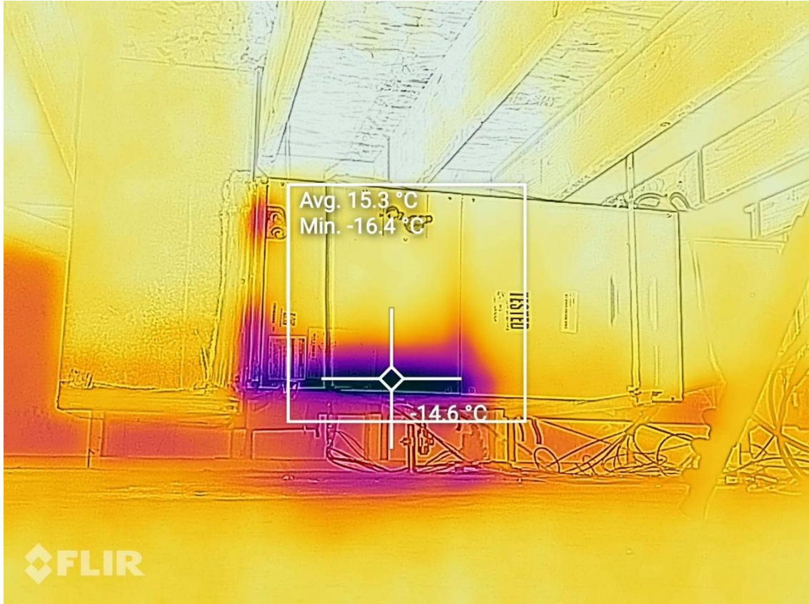
Figure 9 - Thermal Image 1 min into the release
