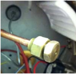
Figure 4.15: Flare fitting 3/8 under test.
