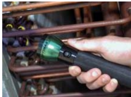
(b) Leak detection by UV torch
