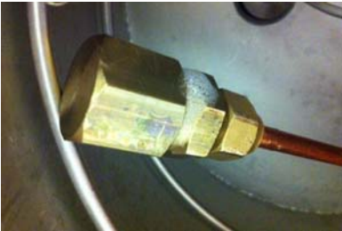
Figure 4.16: Flare fitting 1/2 under test.
